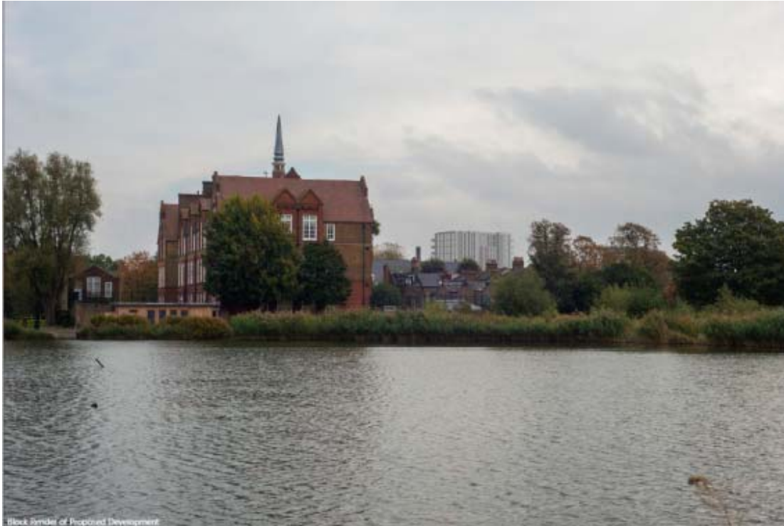
Figure 31. View from Burgess Park across the Cobourg Road Conservation Area.
