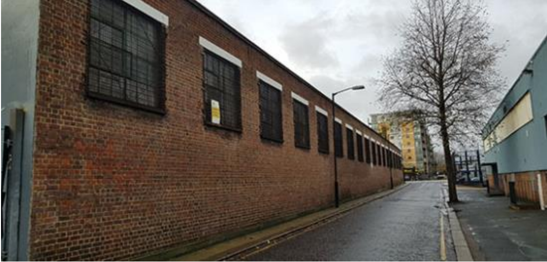
Figure 2. Photograph of site along Bianca Road, retained brick elevation.
